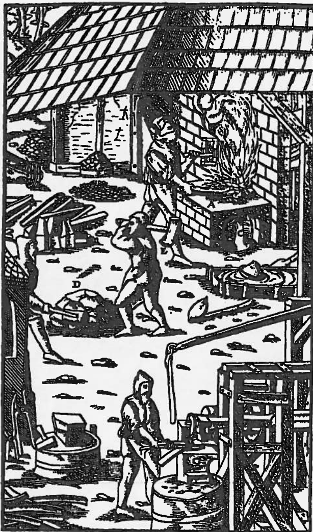
Figure 17. Iron-smelting furnace and forge, mid-sixteenth century.
